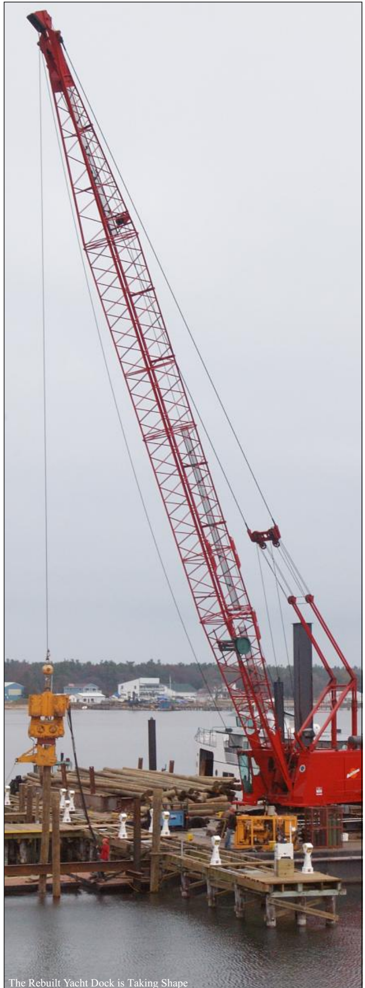
The Rebuilt Yacht Dock is Taking Shape
